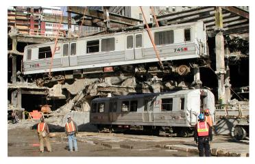
On February 22, 2002, after presenting a plan and getting approval to proceed, two of the PATH cars were extracted and lifted out safely from under the remains of the station. Several weeks later, after completing a structural access ramp down into the site, the two cars were loaded onto low-boy trailers and transported out to Hanger 17 at JFK, where they were stored along with other artifacts from the site.
