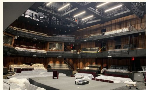
A theater under construction
